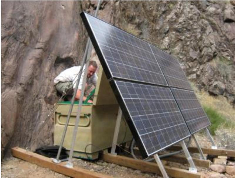
Figure 2. Solar panels and electronics enclosure in Shinumo Creek, Grand Canyon. The Maybell Ditch system will be similar but with fewer panels and the mounting frame will be raised off the ground.
