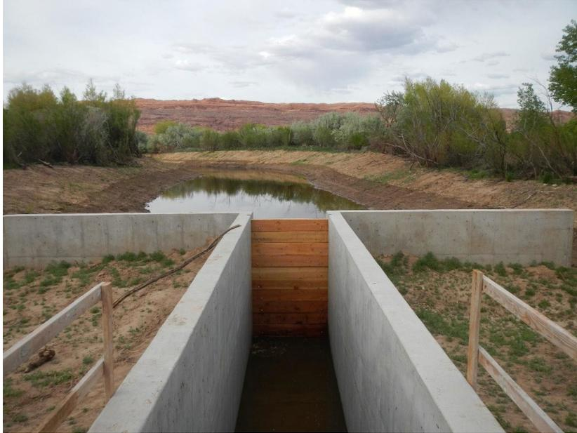
Photo 2. Concrete control structure with stop logs, and newly-excavated “linear pond” where river water & larval suckers will be entrained; view looking inland.
