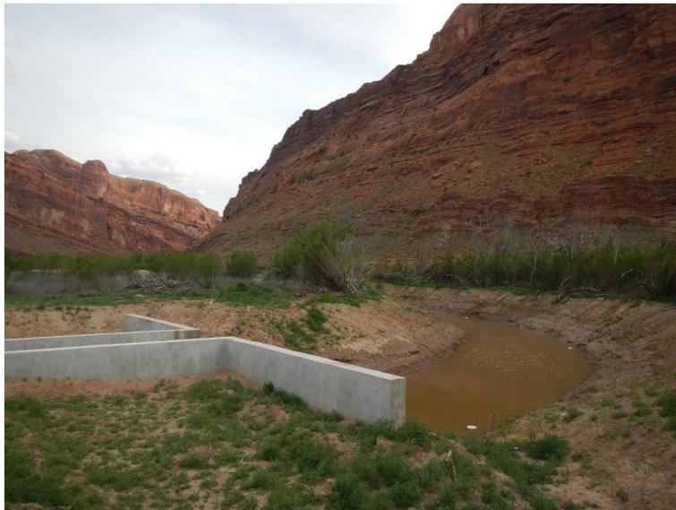
Photo 1. Newly excavated Central Pond inlet channel and concrete control structure; view toward Colorado River, facing slightly downstream.
