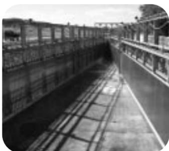
A FISH SCREEN INSTALLED AT THE REDLANDS WATER AND POWER COMPANY DIVERSION DAM AND CANAL BECAME OPERATIONAL IN 2005. THE FISH PASSAGE BECAME OPERATIONAL IN 1996.
