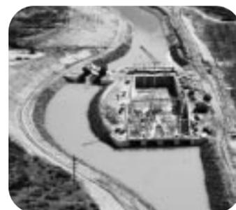
A W-SHAPED FISH SCREEN WAS INSTALLED THIS YEAR AT THE GRAND VALLEY PROJECT DIVERSION DAM AND CANAL. CANAL CHECKS BECAME OPERATIONAL IN 2002, AND A FISH PASSAGE COMPLETED IN 2005 WILL BECOME FULLY OPERATIONAL UPON COMPLETION OF THE PRICE-STUBB FISH PASSAGE IN 2007.
