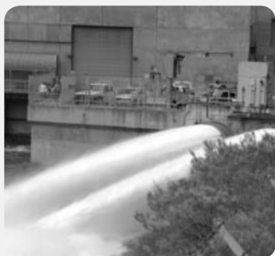
AT FLAMING GORGE DAM WATER RELEASES THROUGH TUBES THAT BYPASS THE POWER PLANT MAY BE NEEDED TO HELP ACHIEVE FLOW CONDITIONS FOR ENDANGERED FISH AS DESCRIBED IN THE RECORD OF DECISION.
