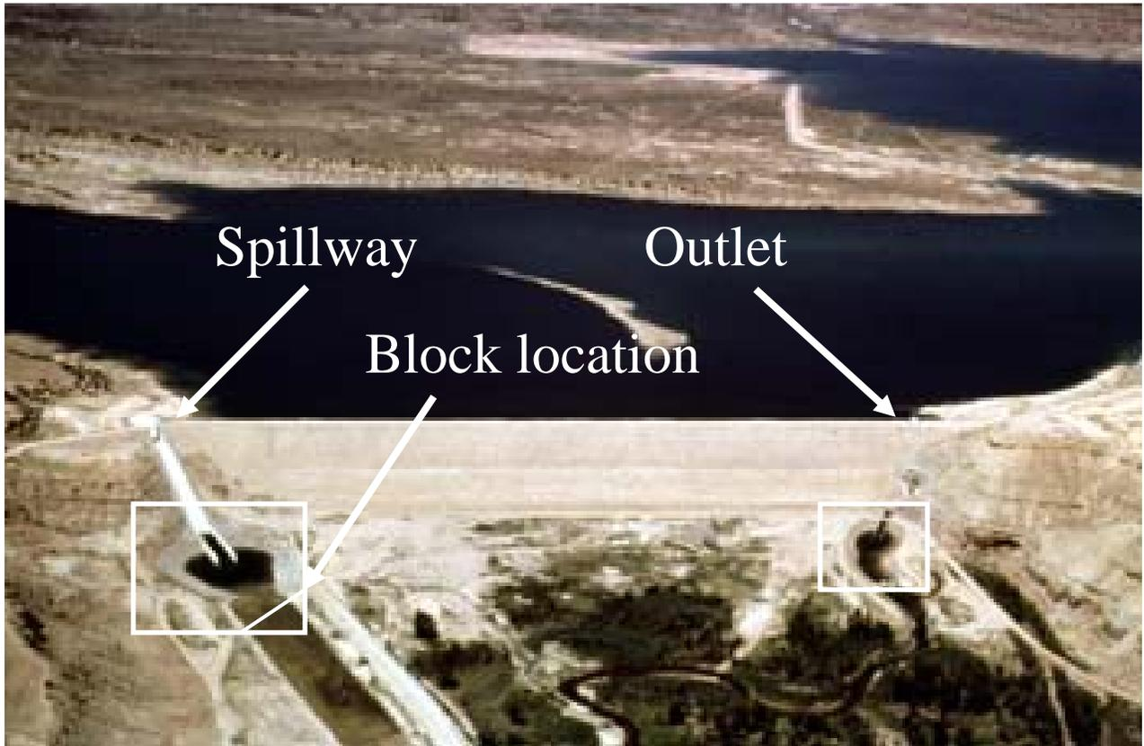
**Figure 2 – Starvation Dam and the spillway and outlet locations. The stilling basins are each identified by a white box. Please note that the outlet is a bottom release of water and the spillway spills water from the top of the reservoir. The block net weir was set below the spillway basin, between the stilling basin and the river.**
