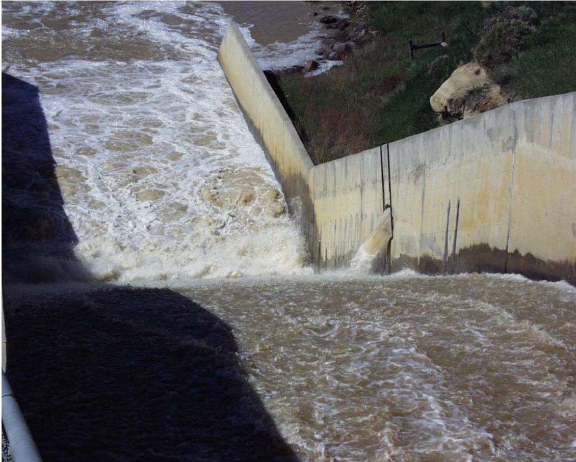
**Figure 4. View of outlet net and spillway.**
