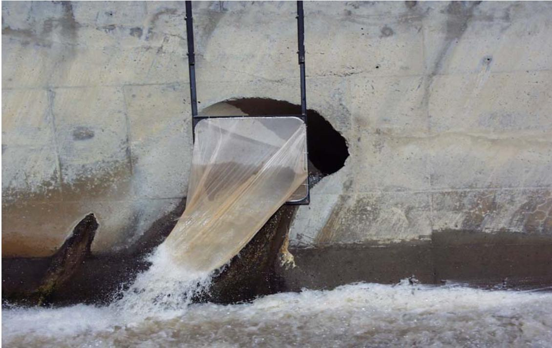
**Figure 5. Elkhead Reservoir outlet capture net.**
