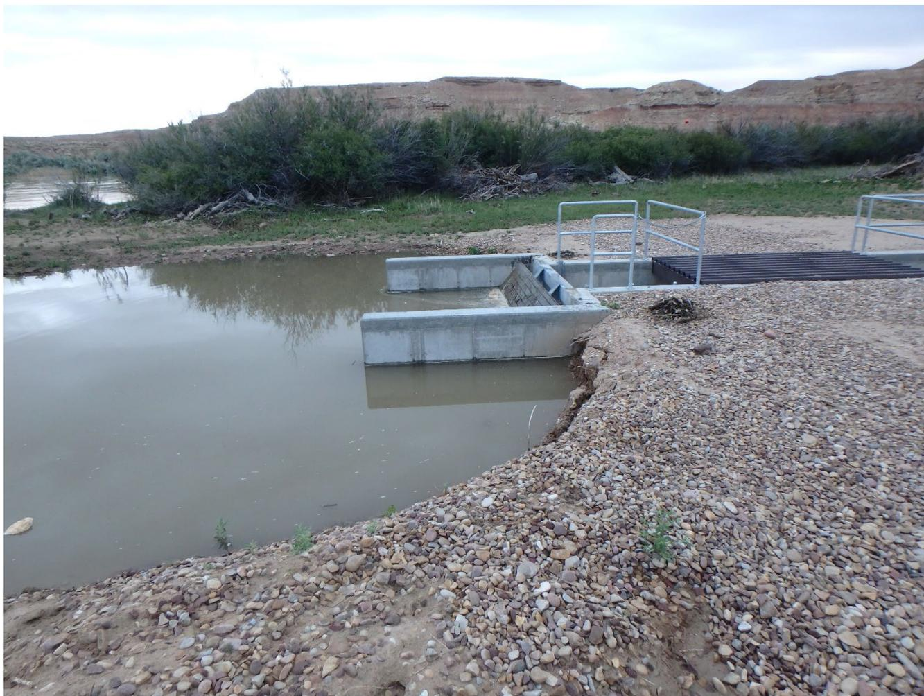
**Figure 3.** Erosion on riverside of the Stirrup wetland water control structure.
