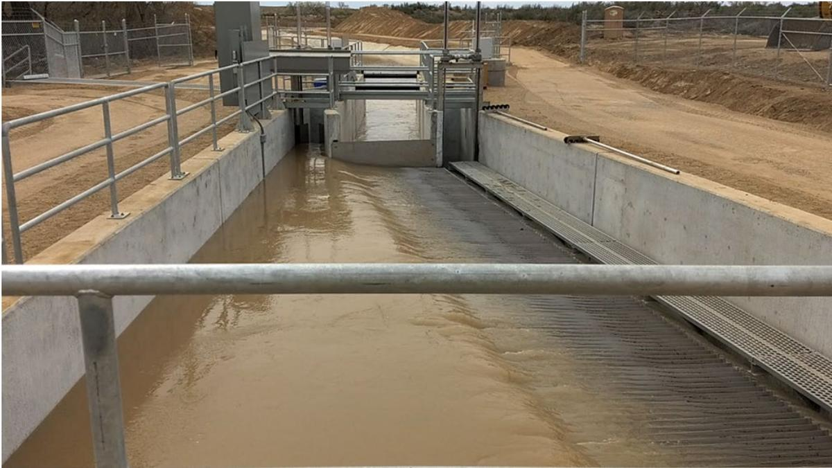
Figure 1. Green River Canal fish screen in operation, looking downstream. Water flows left to right over the screen (foreground right). Screened water drops into the canal entrance while fish and unscreened water is collected and diverted back to the Green River. Note the gap above downstream end of screen, which could allow jumping fish a means enter the canal. Photo: Ryan Christianson
