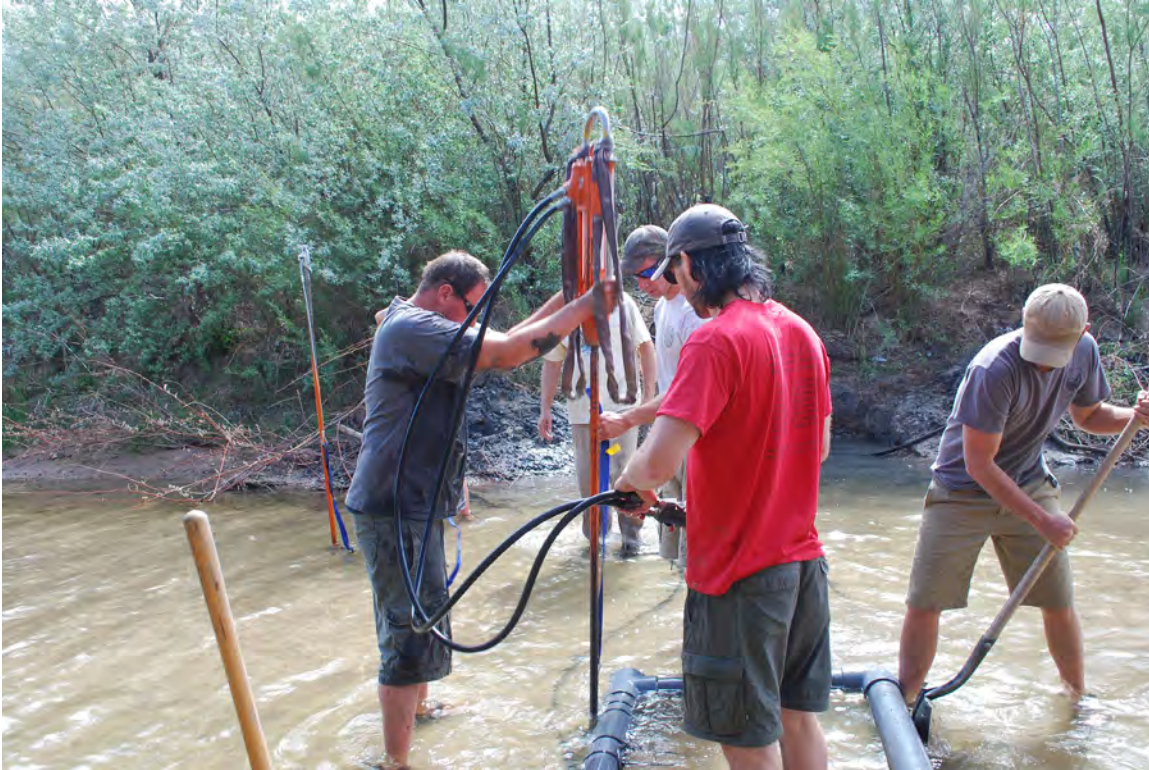
Figure 2. Anchoring the antenna using duck-billed anchors and a hydraulic hammer.
