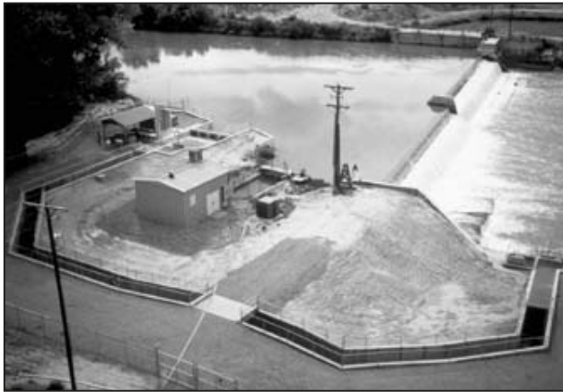
The fish ladder at the Redlands Diversion Dam on the Gunnison River is operated to share water shortages while providing fish passage.
