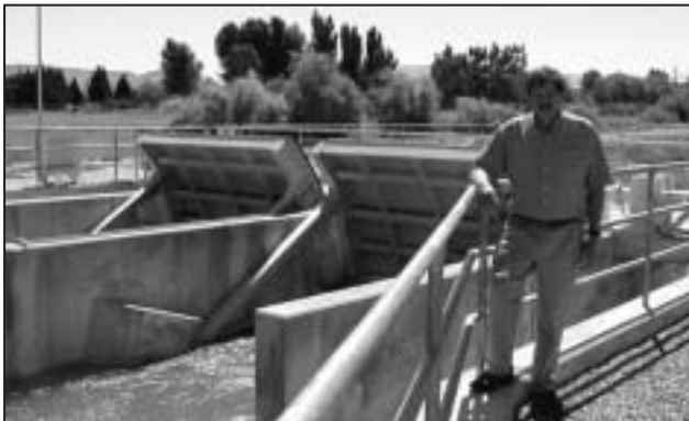
U.S. Fish and Wildlife Service Hydrologist George Smith assisted in development of the Grand Valley check structures which have allowed water users to make more efficient use of limited water resources. "Saved" water is available to increase river flows for the endangered fish.
