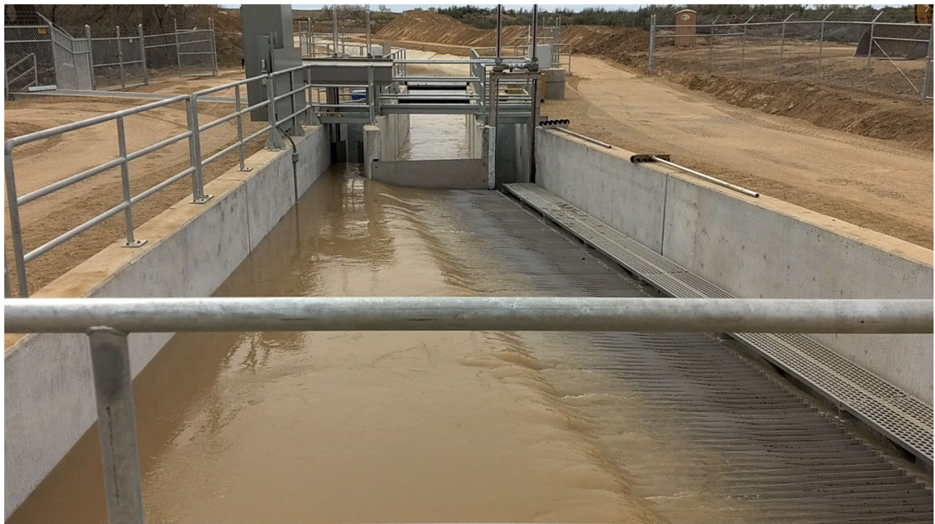
Figure 2. Green River Canal fish screen in operation, looking downstream. Water flows left to right over the screen (foreground right). Screened water drops into the canal entrance while fish and unscreened water is collected and diverted back to the Green River. Photo: Ryan Christianson, USBR.
