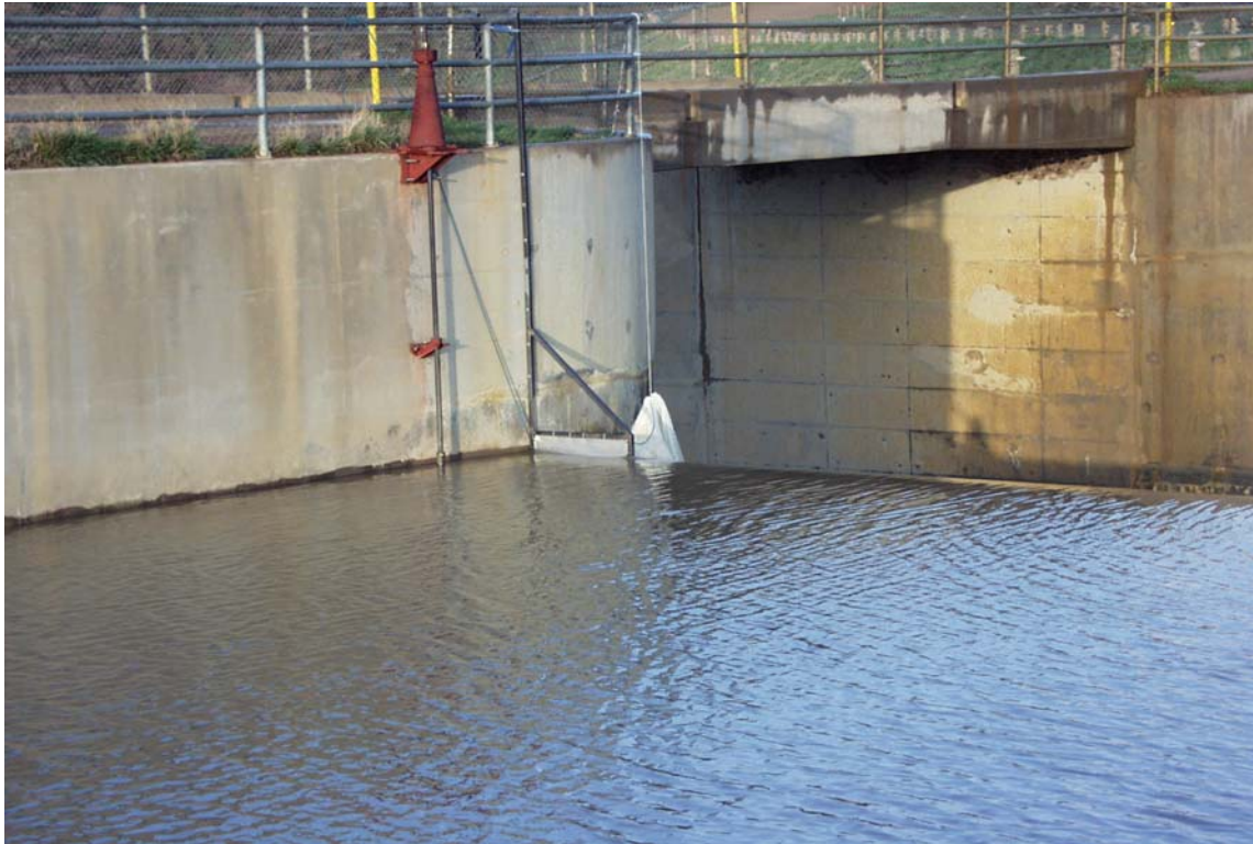
Figure 2. Net on edge of spillway.
