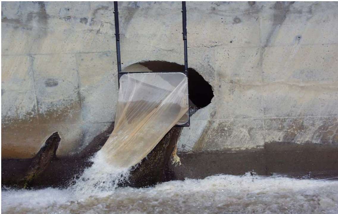
Figure 1. Elkhead Reservoir outlet capture net.
