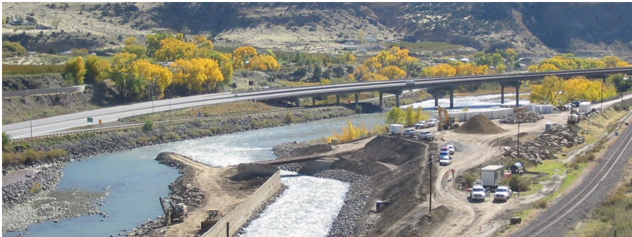
Photo 15. Price-Stubb fish passage construction. Photo credit USFWS.
